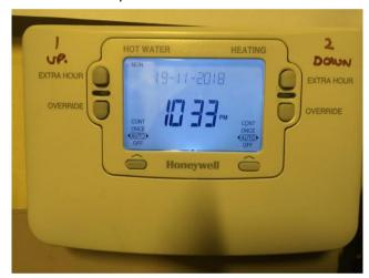
The LH Channel controls the heating upstairs and the RH channel controls the heating downstairs.
